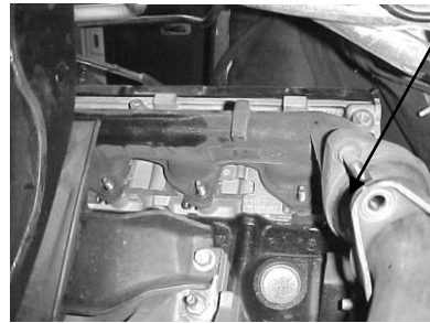
#6 . FACTORY FLANGE CONNECTION . DISCONNECTING POINT .
